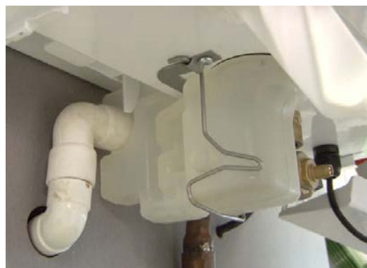
Figure 3 General Access - Location of condensate trap and retaining clip
