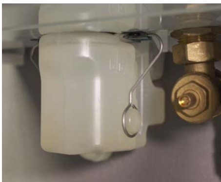
Figure 3 General Access - Location of condensate trap and retaining clip
