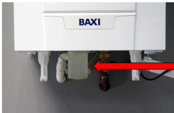
Figure 3 General Access - Location of condensate trap and retaining clip
